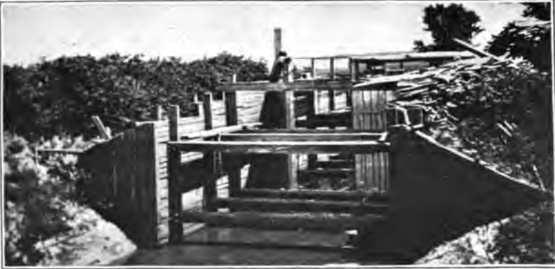
FIG. 1.—WOODEN OUTLET IN HARTWELL RANCH LEVEE.
