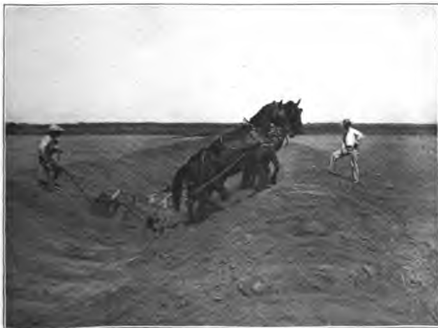
FIG. 2.—CONSTRUCTING LATERAL DITCH WITH SCRAPER.
