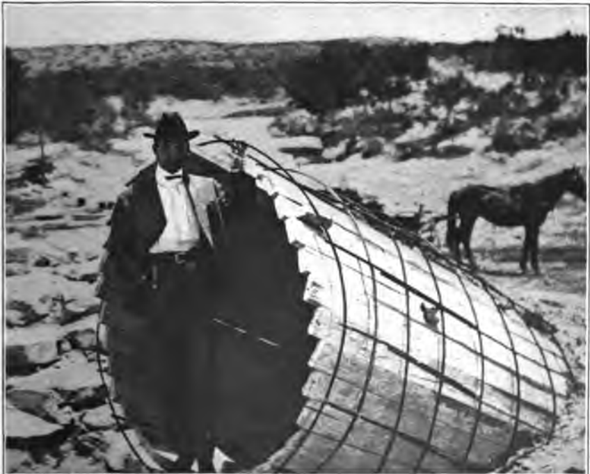
FIG. 2.—DEL RIO CANAL, TEXAS. REINFORCED CONCRETE PIPE IN COURSE OF CONSTRUCTION.
