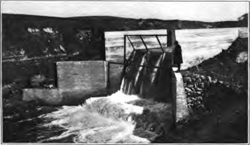
FIG. 1.—A 15-FOOT CONCRETE DROP ON MODESTO CANAL.
