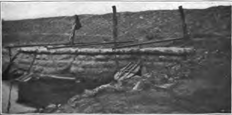
FIG. 3.—OUTLET END OF OUTFLOW CULVERT IN FLINT CREEK-IOWA RIVER LEVEE, SHOWING METHOD OF COUNTERBALANCING CAST-IRON VALVES.
