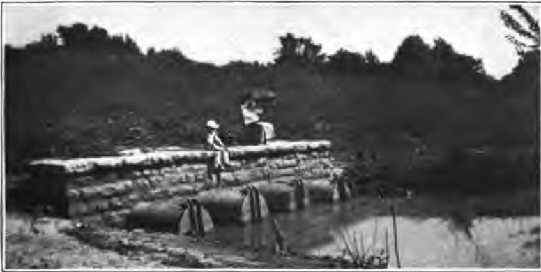
FIG. 2.—OUTLET END OF OUTFLOW CULVERT IN FLINT CREEK-IOWA RIVER LEVEE, SHOWING WOODEN VALVES.
