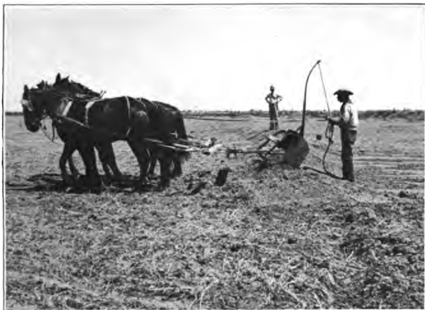
FIG. 1.—CONSTRUCTING CHECK LEVEE WITH SCRAPER.
